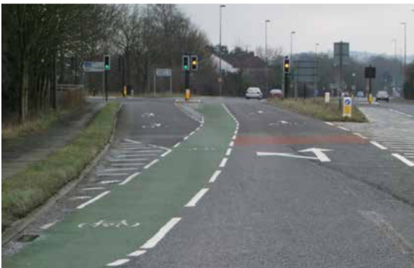
Use of dashed lane markings and surface colour to highlight a cycle lane to motorists seeking to enter a left-turn lane
